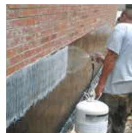
For fast, easy foam board installation, simply spray and stick with 3M™ HoldFast 70 Cylinder Spray Adhesive. Bonds foam to concrete, waterproofing, OSB and more without damaging the foam.
